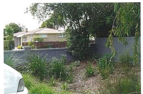
This swale designed to manage stormwater from the car park is planted with native species which thrive in boggy areas, such as astelia, flax, toi toi, empodisma, manuka, carex, and ti kouka (cabbage trees).
